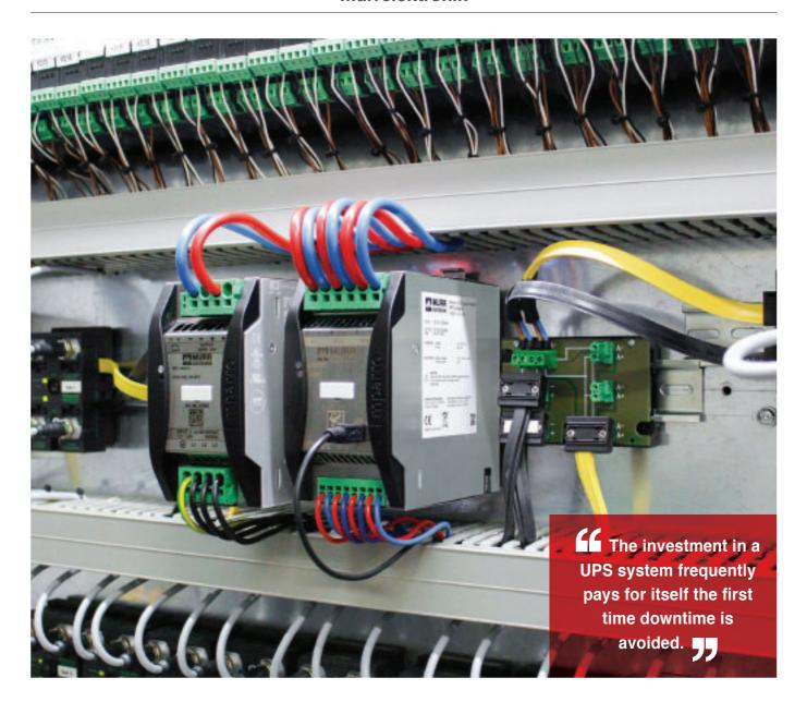
ew things are as irritating (or as expensive) as unplanned downtime in plants and machines. The Murrelektronik UPS module Emparro ACCUcontrol extends the high-performance Emparro power supply system and keeps machines running by switching smoothly to battery operation in the event of a mains power failure. The investment in a UPS system frequently pays for itself the first time downtime is avoided.
